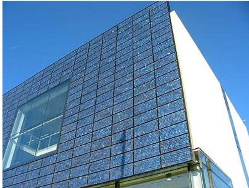
Figura 4.9: Manchester College of arts and technology, Manchester Fuente: Cortesía de SolarCentury.com
